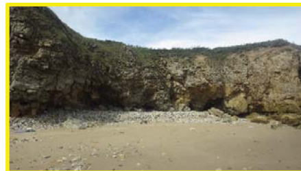
Further rockfalls within the harder rock cliff.
