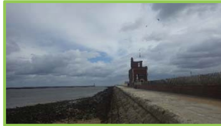
Minor re-pointing and repairs to South Pier.
