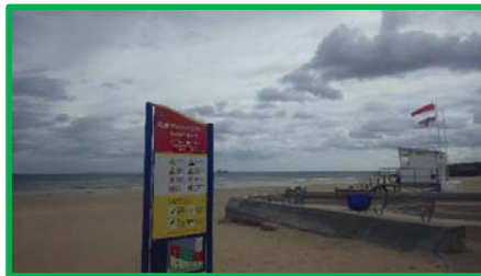
New concrete wall at the lifeguard station.
