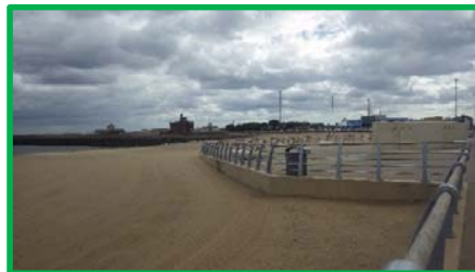
Southern section of new seawall promontory.
