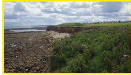
Small localised slumps at southern section of rifle ranges.
