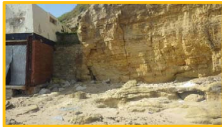
Cracking of cliff face and undermining of structure at north end of Marsden Bay. Voids in cliff face.
