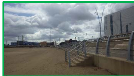
Southern section of new seawall.
