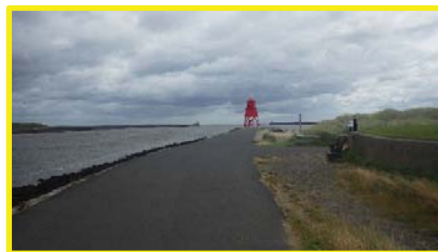
Resurfacing of the bitmac deck of the South Groyne.
