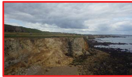
Recent rock falls in cliffs at Lizard Point Carpark.
