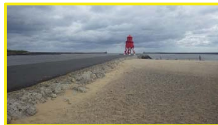
Cracking and onset of voiding in concrete on south facing side.
