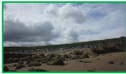
Rock revetment in very good condition.
