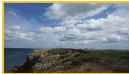
Recent slumps in overlying soft material.
