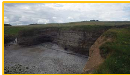
Slippage of soft material at Potters Hole.
