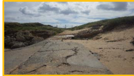
Breaking up of ramp at south end of dunes.
