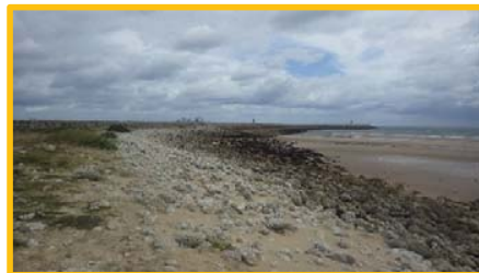
Cobble berm at northern section of Sandhaven.
