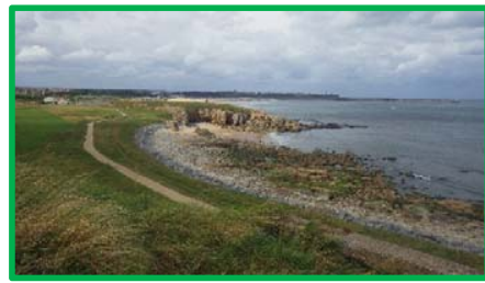
Graded slope in very good condition
