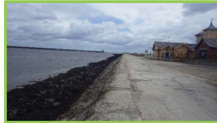
Minor re-pointing and repairs to South Pier.
