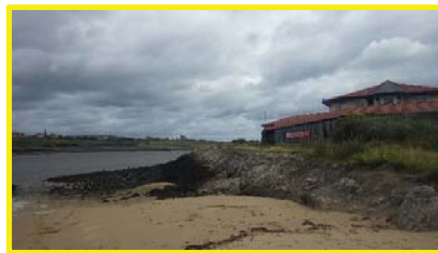
Grouted masonry revetment on south side of wave basin.
