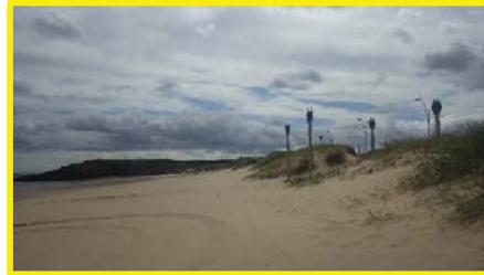
Narrow dunes burying gabions at southern end of Sandhaven.
