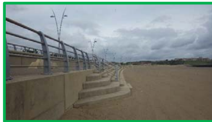
Northern section of new seawall at Littlehaven.
