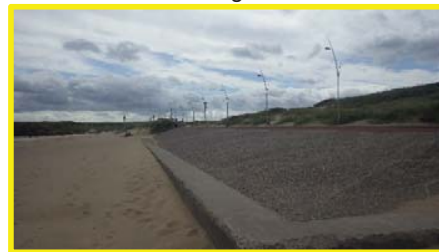
Minor settlement to revetment but no cracking visible.
