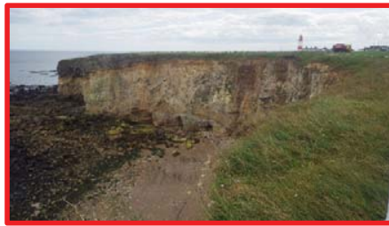
Cliff failure in cliffs fronting Lizard point Car Park.
