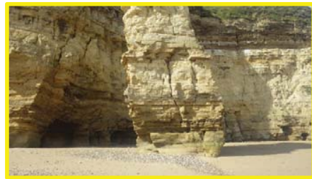
Cave formation and vertical cracking in Lot's Wife stack.
