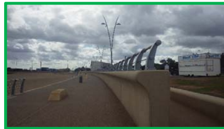
Setback crest wall along northern section of new seawall.
