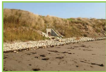
Outfall has been reconstructed at south end of frontage.
