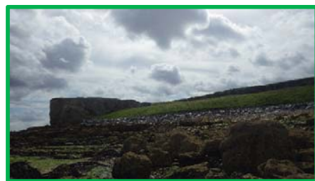
Rock revetment and re-graded slope in very good condition.
